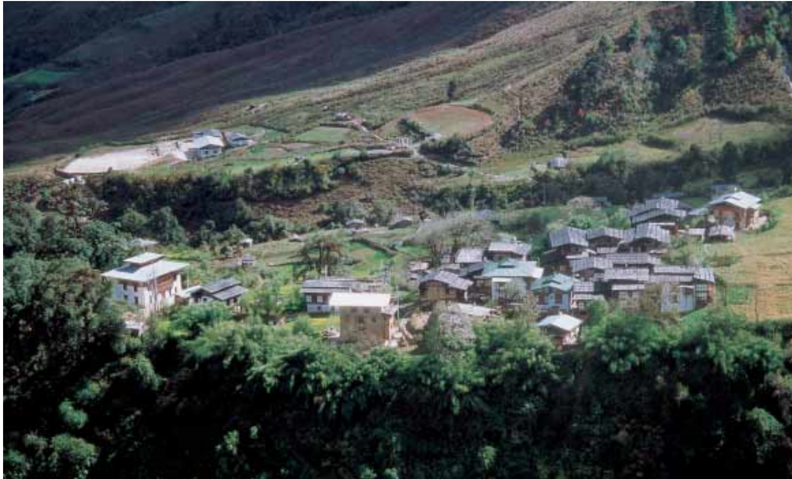
Rukubji: spatial configuration 1994: demolition and re-erection as strategy for mediation in the conflict
