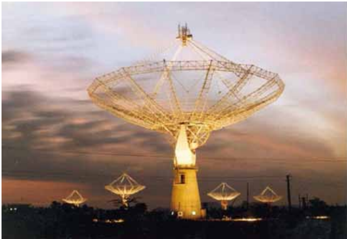
Figure 1: GMRT consists of 30 individual 45 meter dish antennas, with a collecting area of nearly 50 000 m 2 . The array is spread over a distance of 25 km, arranged in a Y pattern for the outlying arm antennas, and a concentration of 12 antennas in a central square.
