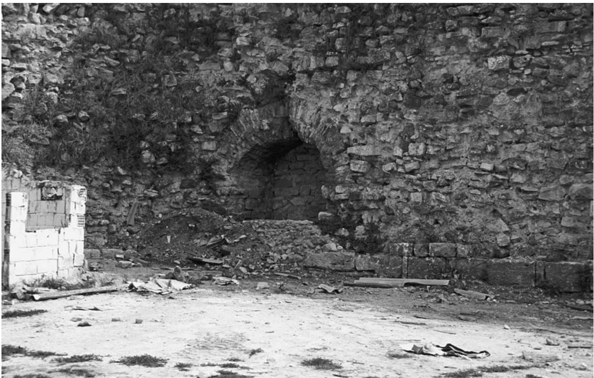
110 Metrai (Çatalca), N-Mauer, Detail
