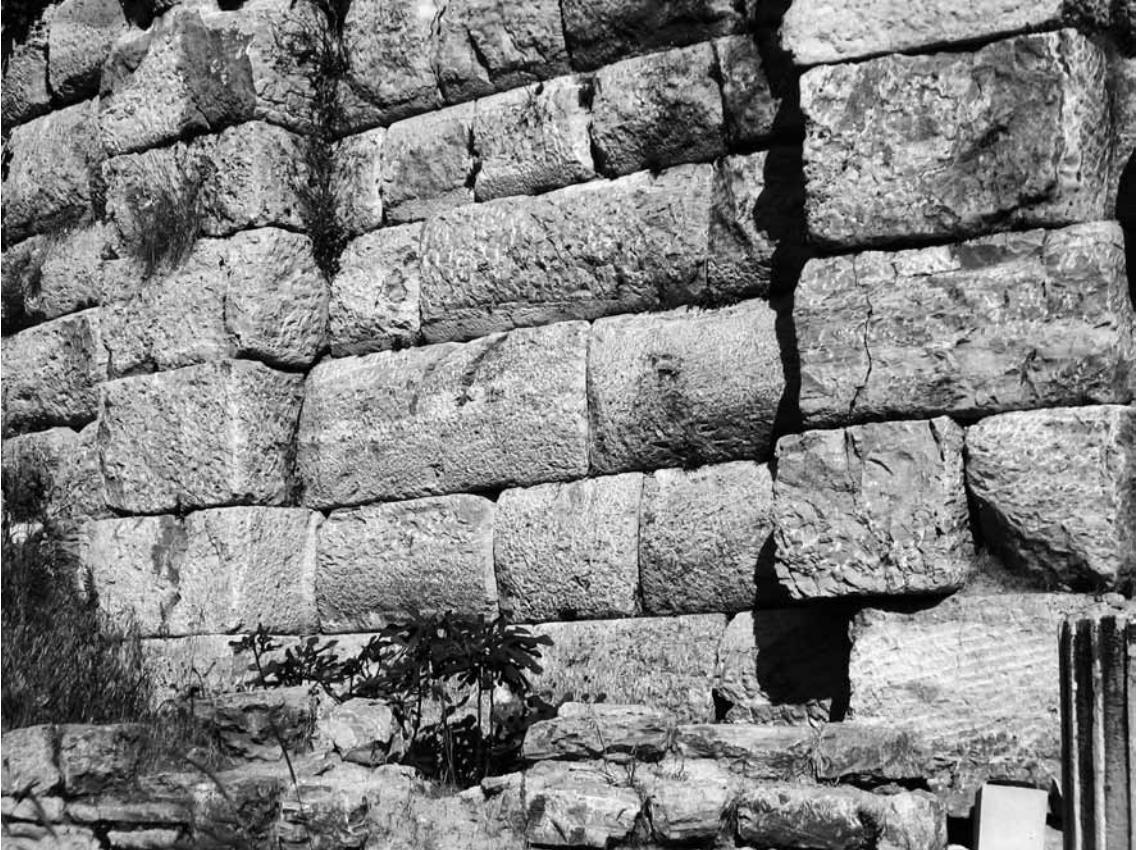
2 Retaining wall, detail between buttress 2 and 3
