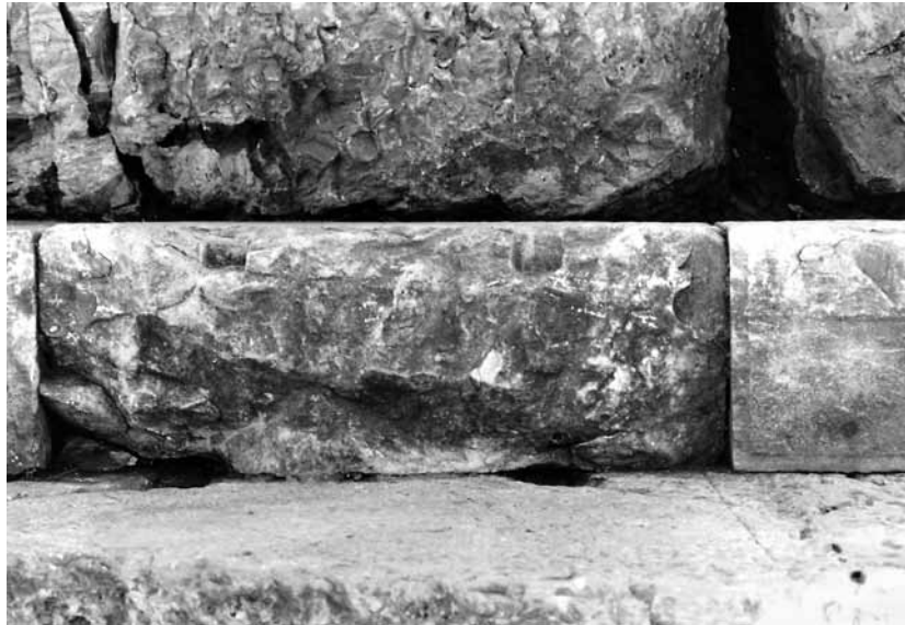
1 Remains of pilaster base on footing of rear wall
