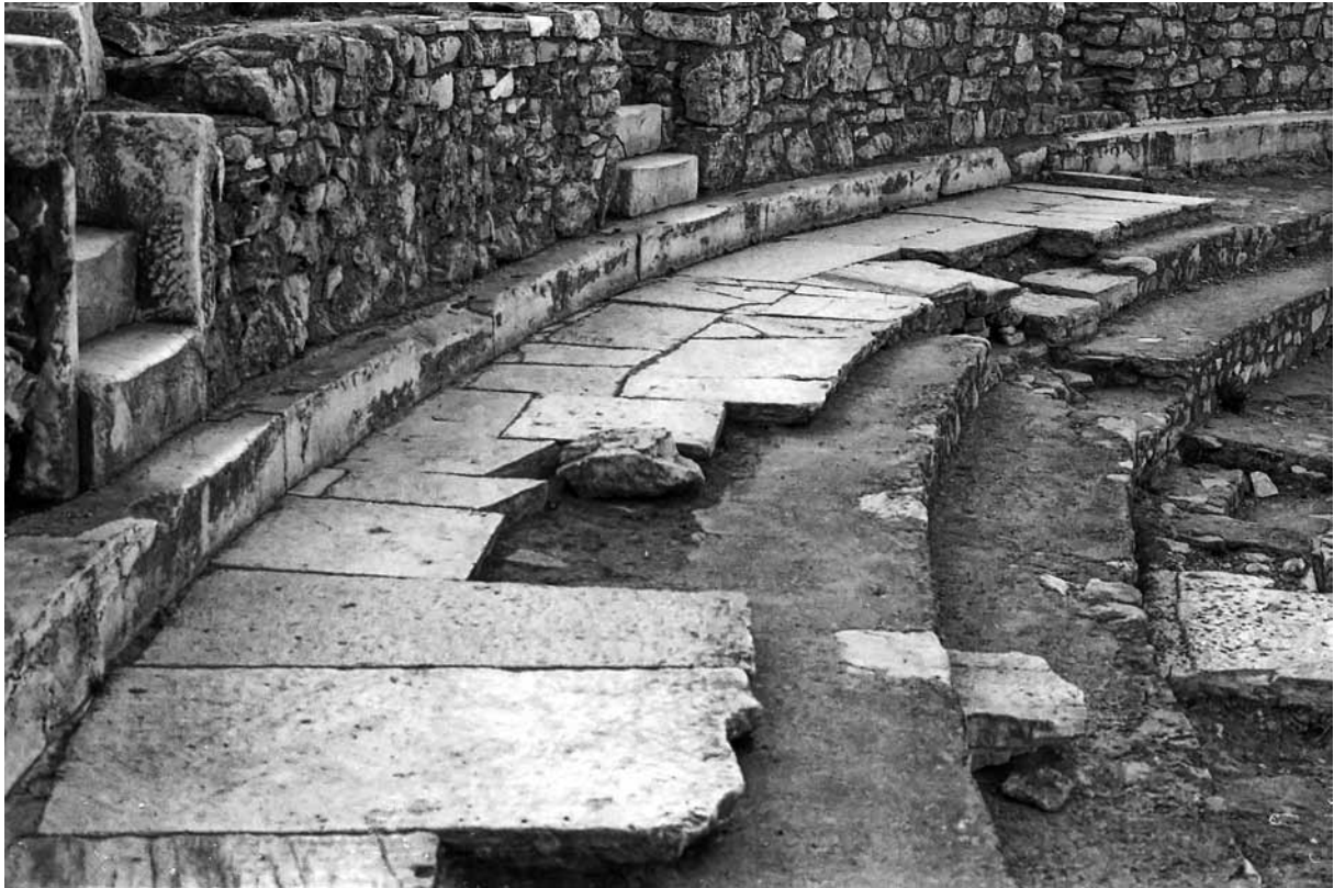
1 Paving of the middle diazoma
