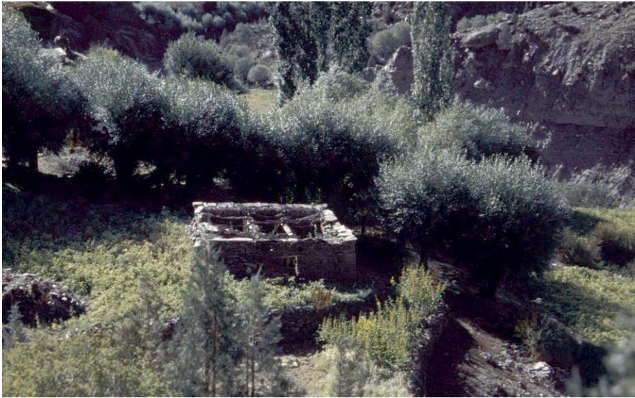
Figure 7.6 Collapsed temple of Johling. Photo: V. Widorn 1998.
