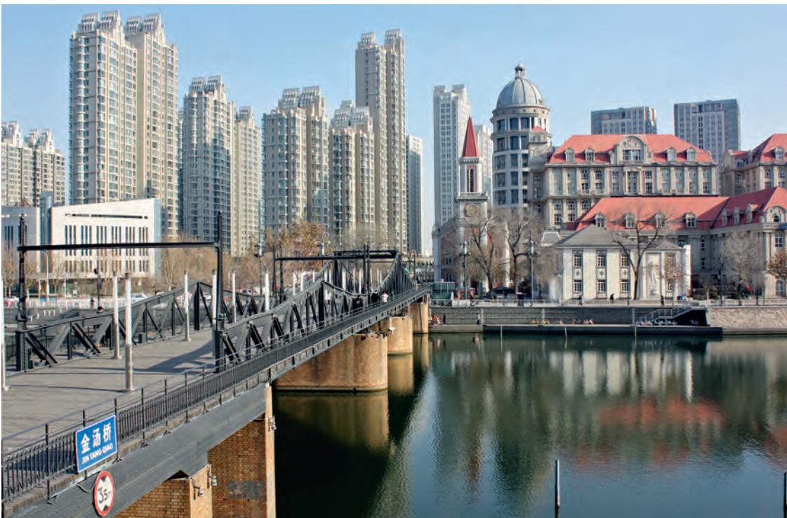
Figs. 78a,b Photographs taken by Michael Falser in Tianjin in December 2018 in the former Austro-Hungarian concession: Above: A view from the north-west of the former 'Chinese' side across the river towards the former Austro-Hungarian concession: the surviving 'Austrian Bridge' stands in the middle ground and the concession itself in the background to the left-hand side. Below: A view across the 'Austrian Bridge' towards the former Austro-Hungarian concession; its former, white consulate building is in the background to the right-hand side.
