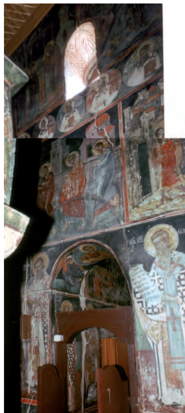
Fig. 17 Basilica of Dormition, Kalampaka, Thessaly, South wall of the Holy Bema where the joint can be distinguished
