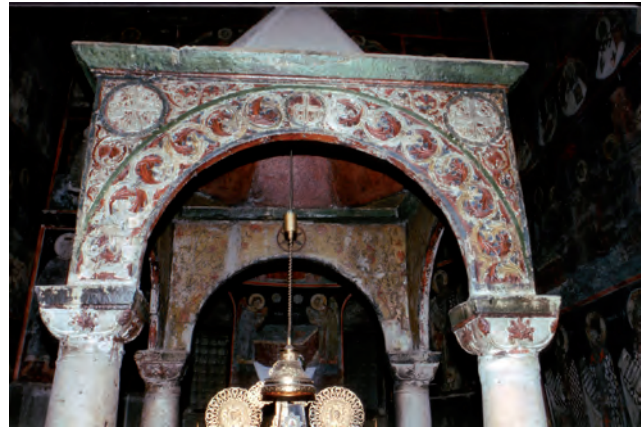
Fig. 30 Basilica of Dormition, Kalampaka, Thessaly, West elevation of the ciborium
