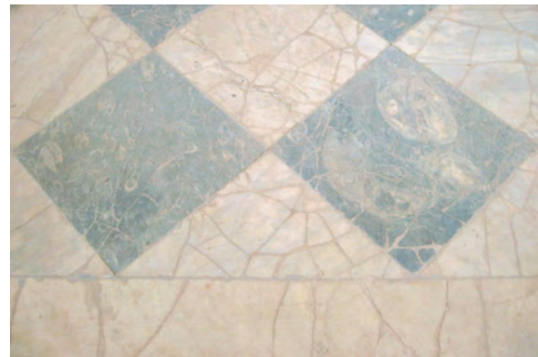
Abb. 2: SR 22/23: Bodenbelag, Detail
