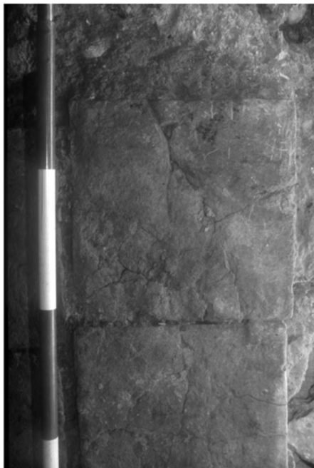
Abb. 17: SR 30, Ofen 6, Detail Bodenplatten
