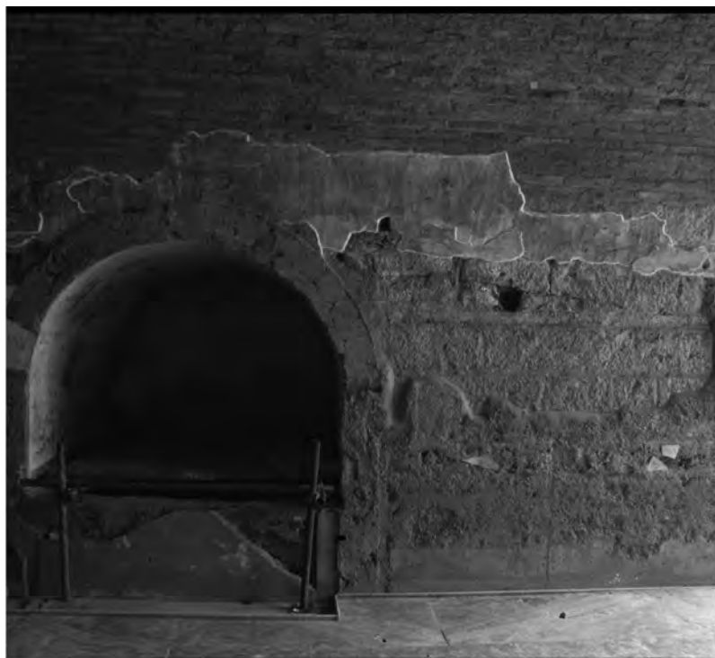
Abb. 6: Raum 36a, N-Mauer
