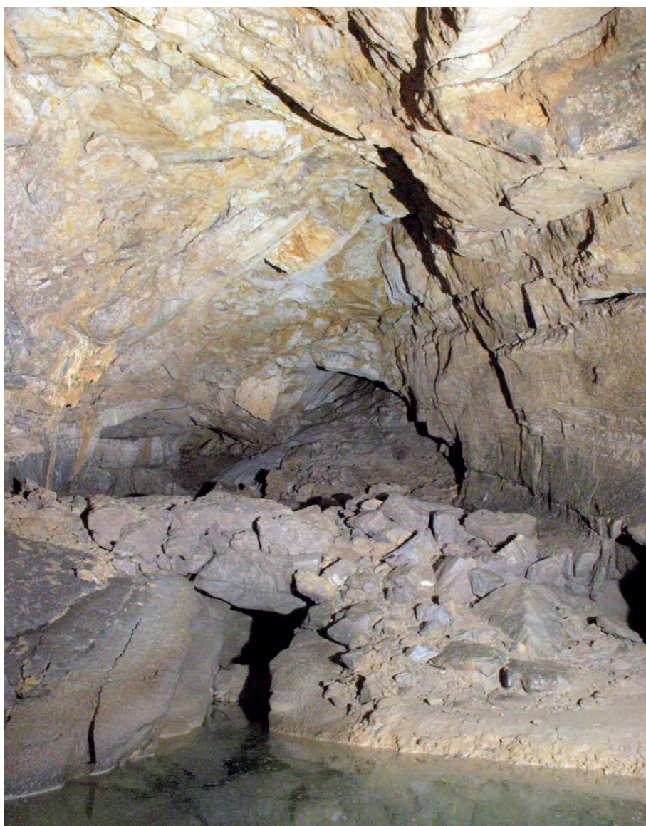
Figure 4: Collapsed zone above 2 nd lake in Križna jama.
