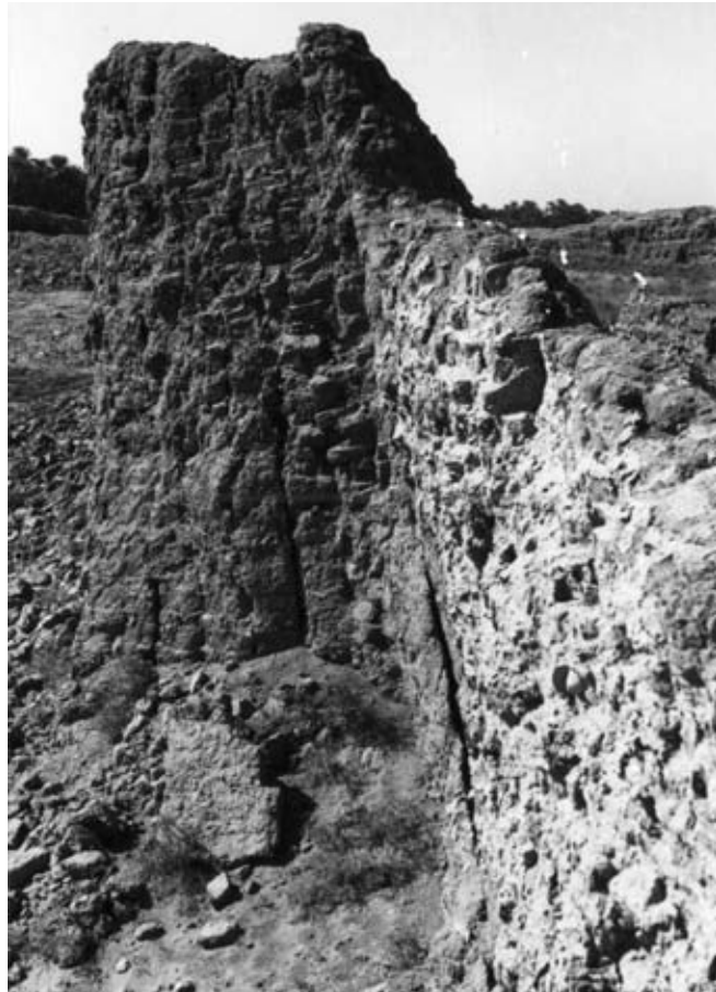
Fig. 15 Construction in vertical layers of inner wall of Double Walls (situation in 1966, photo CFBE)
