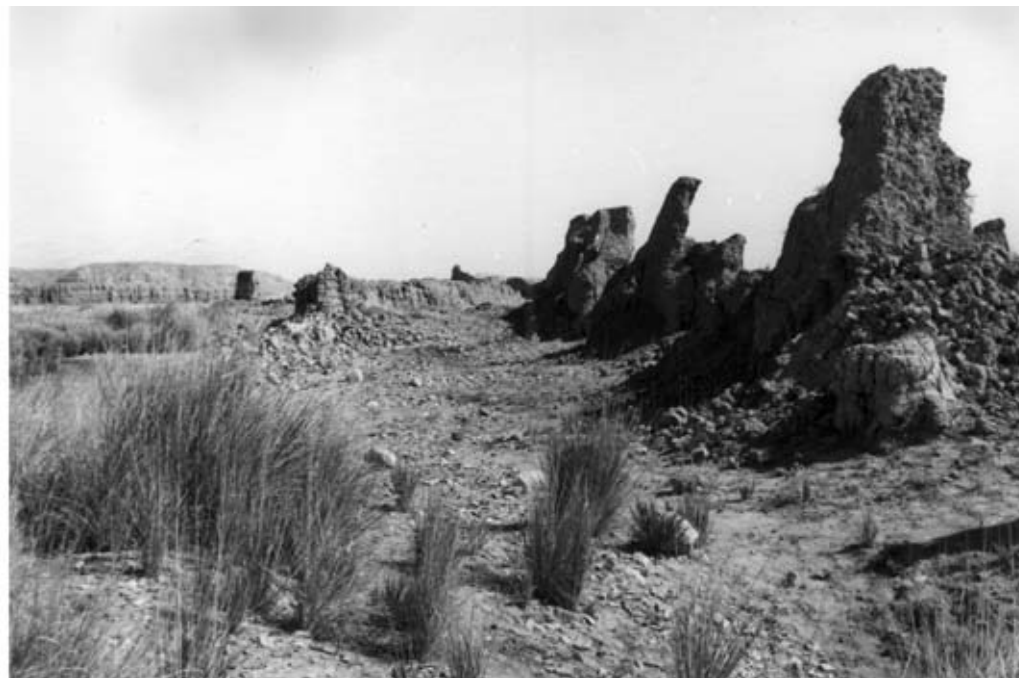
Fig. 16 The Double Walls; inner wall at right side (situation in 1966, photo CFBE)
