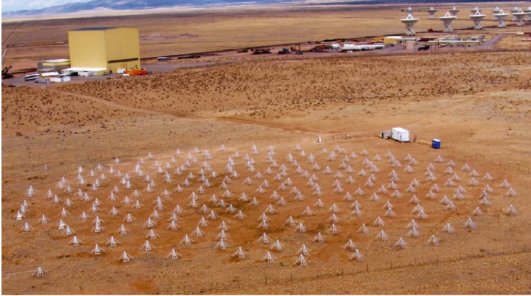
Figure 1: The 256 dual-polarization dipoles of the LWA1 are seen in the foreground with the associated electronics shelter to the right of the station and the National Radio Astronomy Observatory's Jansky Very Large Array in the background (reproduced with permission from Greg Taylor).
