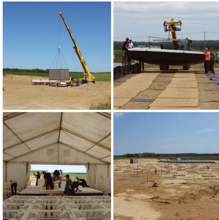
Figure 5: The LOFAR station in Baldy under construction.
