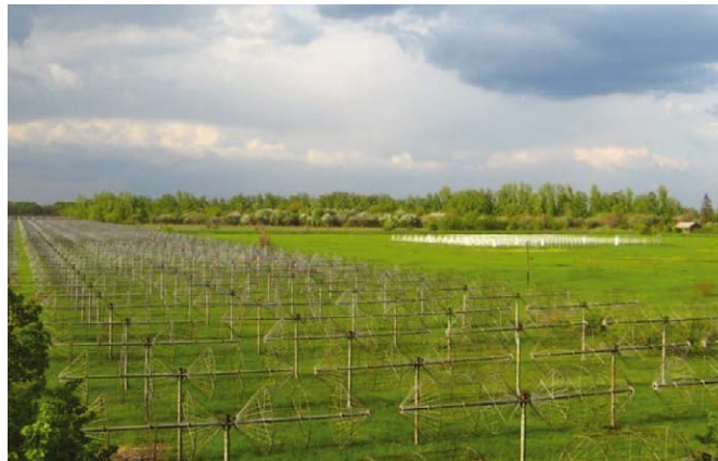
Figure 7: North-south arm of the radio telescope UTR-2 (foreground) and the radio telescope GURT behind it (white color).
