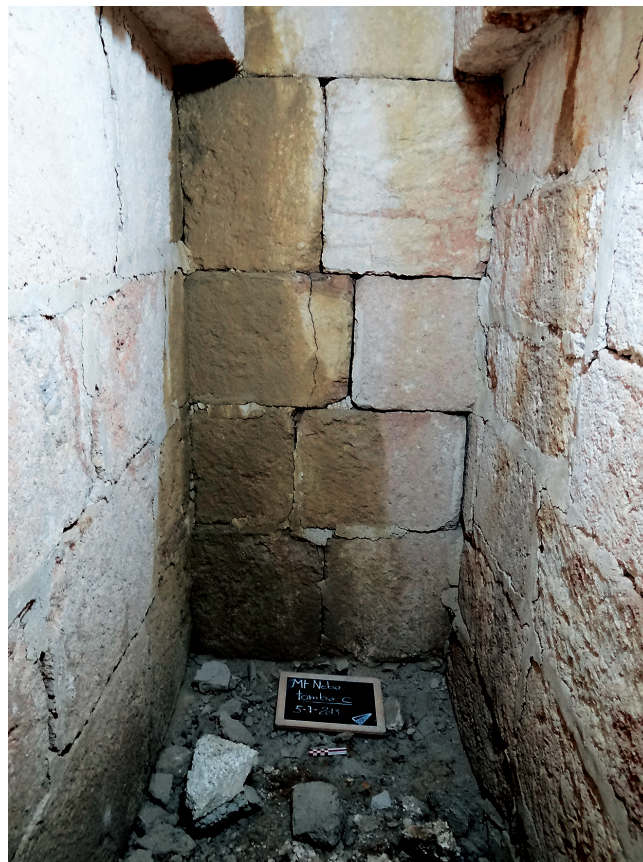
Fig. 55 Memorial of Moses. Interior masonry of the tomb no. 73.
