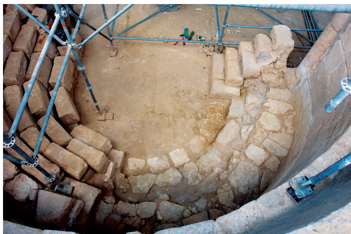
Fig. 16 Memorial of Moses. Presbytery of the Basilica, demolition of the upper rows of the synthronon – layer SU2.
