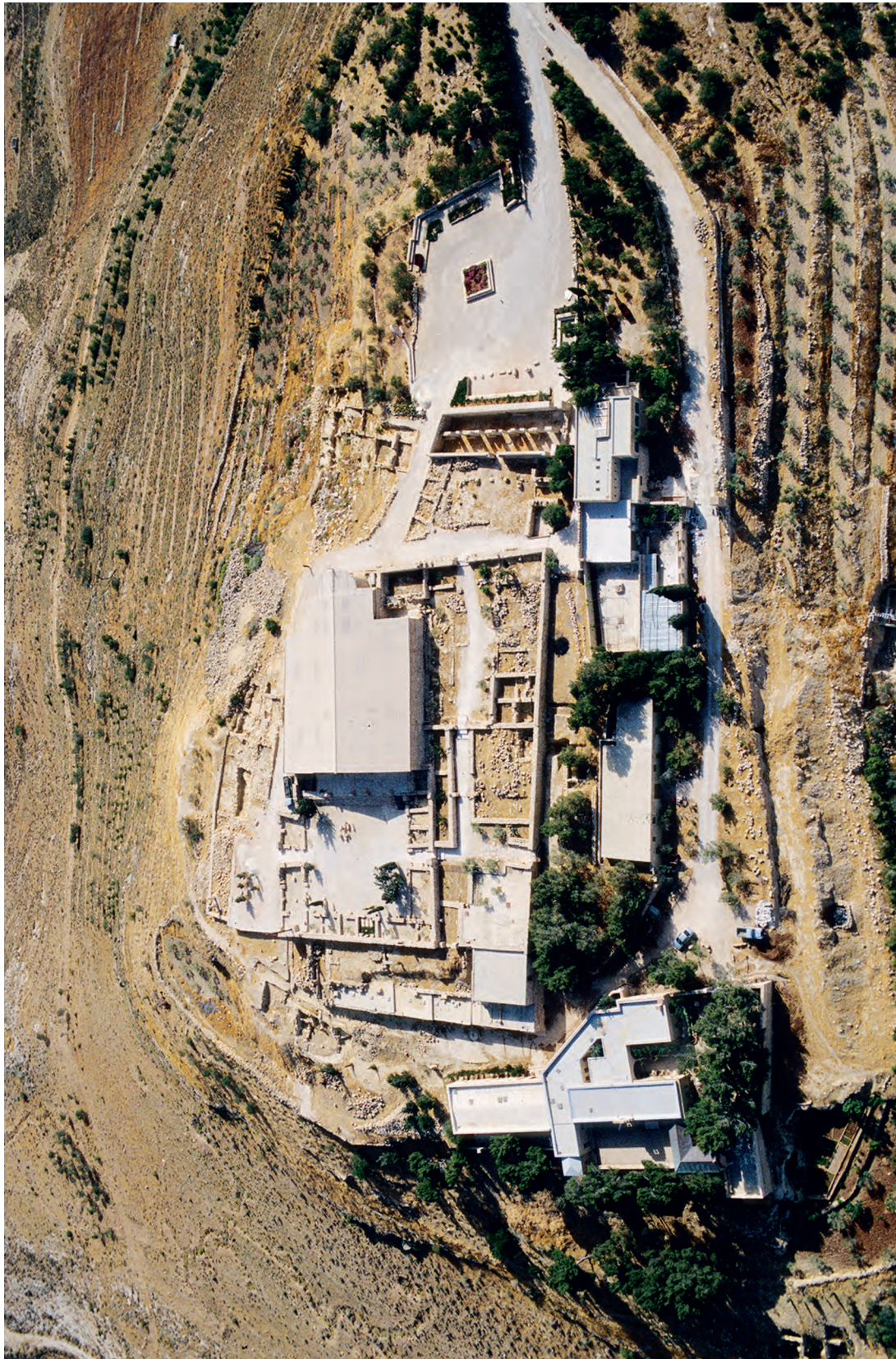
Fig. 140 Memorial of Moses. Aerial photo of the monastic complex (© APAAME).
