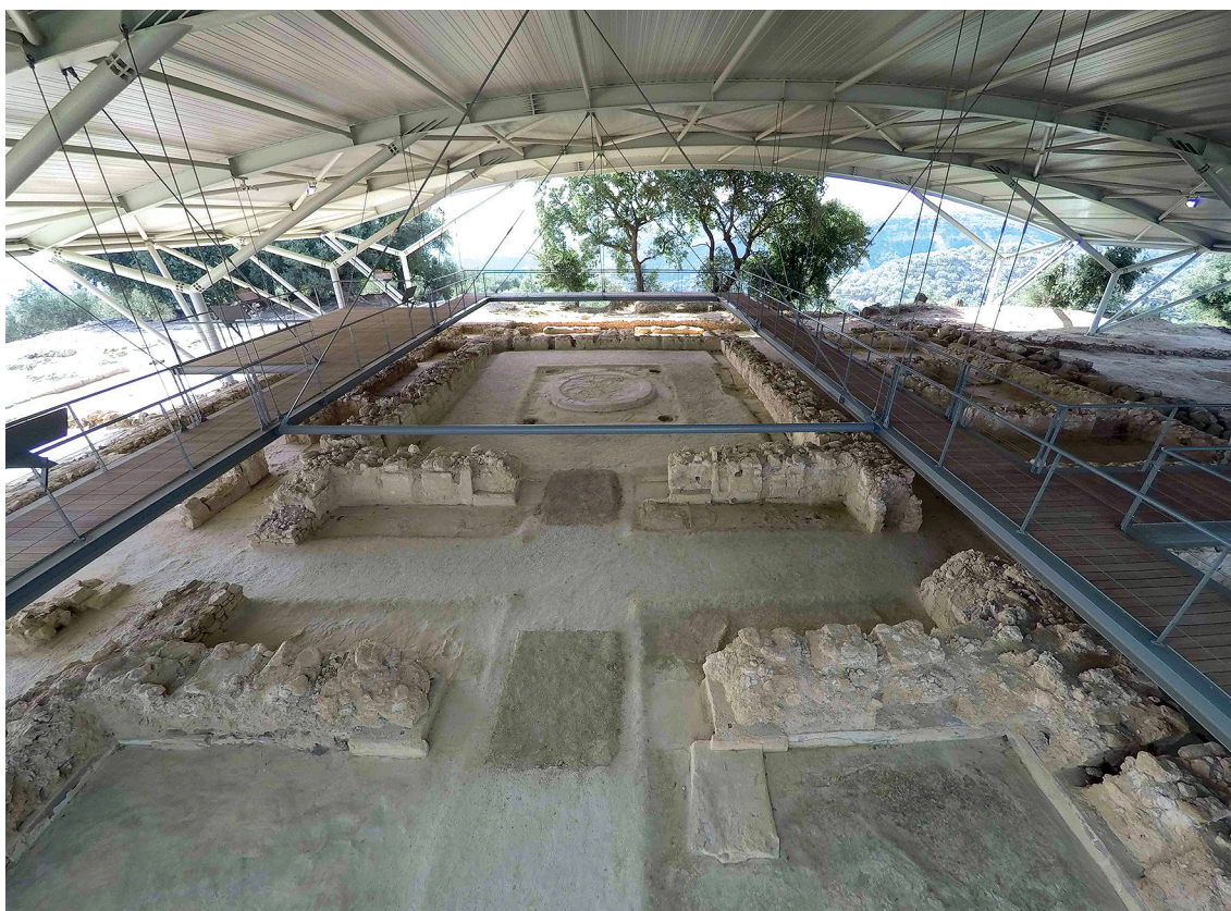
Fig. 2: New shelter over the central corridor of the Palace of Nestor, June 2016, looking northwest (Ephorate of Antiquities of Messenia/Department of Classics, University of Cincinnati)
