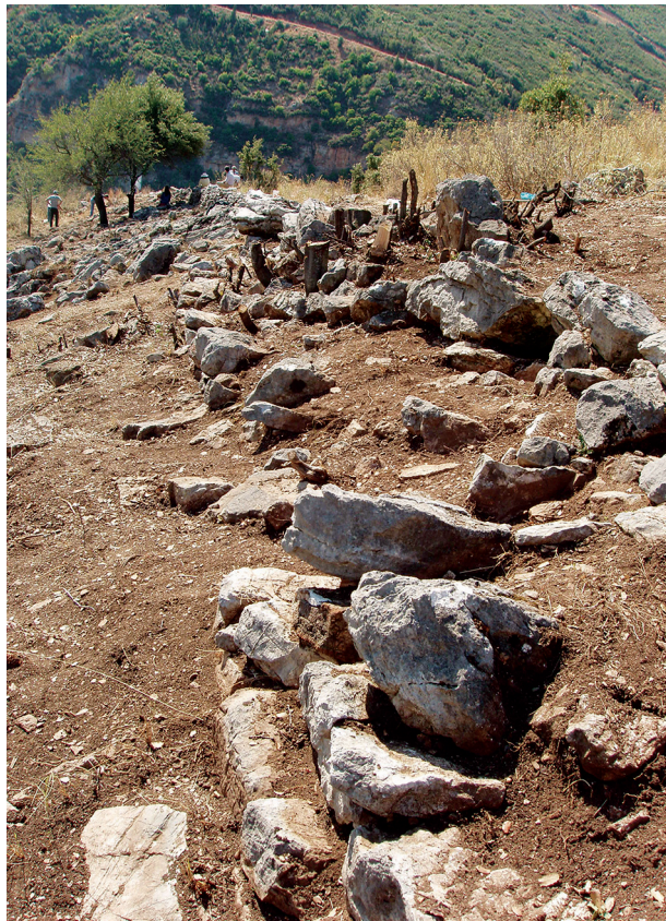
Fig. 4: Exterior face of the wall on Terrace 3 (photo: L. Papazoglou-Manioudaki)
