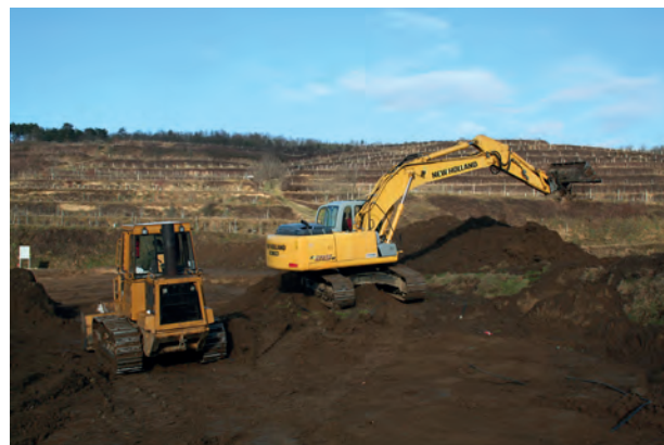
Fig. 6. Kammern-Grubgraben 2015, extensive earthworks to remove the irrigation system northwest of the site on land parcel 430/3 (photo: T. Einwögerer, OeAI, OeAW).
