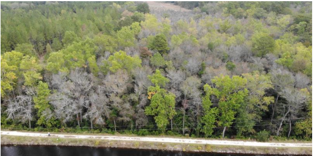
Figure 1: An oblique view of Sweet Bay Pond Dam in Columbia, SC. Photo was taken with a DJI Mavic Pro on October 26, 2019.
