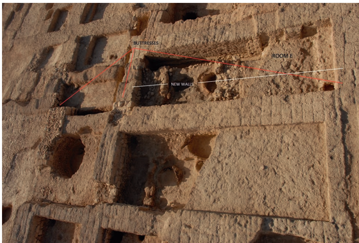
Fig. 3 View of Room E showing the new walls added and the pre-existing buttresses
